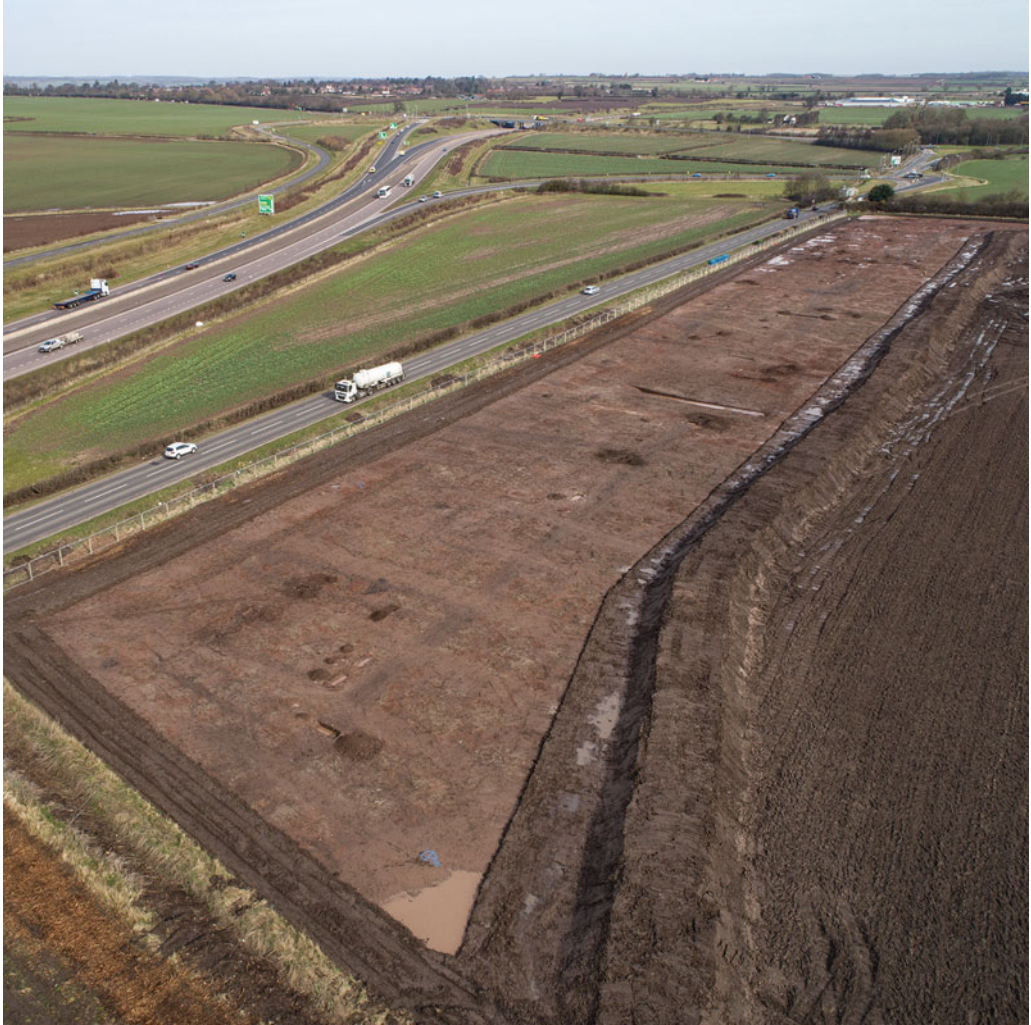
FIG. 2. Aerial view of the Chapel Lane excavation, facing north. The road to the left is the A46 Newark to Widmerpool Improvement Scheme and the road adjacent to the site follows the presumed line of the Fosse Way. Margidunum Roundabout is marked by the trees at the right edge of the view.
