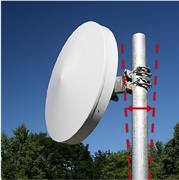
Figure 1. Cassegrain reflector antenna with small boom movements.
