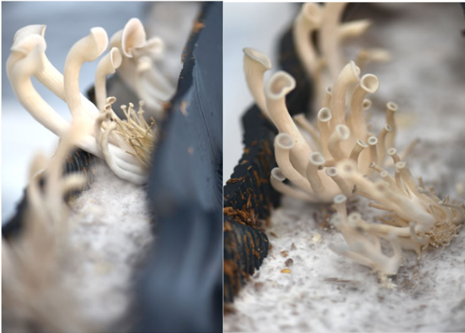
Figure 5. Mycelium growing inside the wall panel system.
