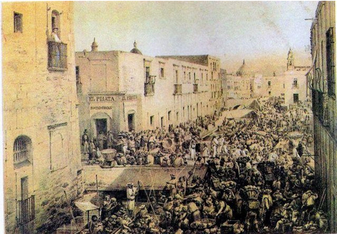
Figure 7. Loading pier of the Calle Roldán, showing the intensity and continuity of traffic between land and water. Boats in the foreground represent lake transport, and a bridge at the back represents land transport. Image from Casimiro Castro and J. Campillo 1864.
