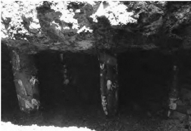
Figure 8. Acequia de La Merced, showing its construction on stilts (Lugo Ramírez 2007).
