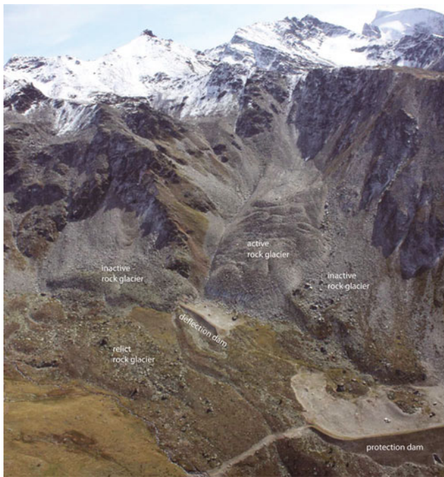
Fig. 8. Avalanche deflection and protection dams constructed in contact with relict, inactive and active viscous flow features of mountain permafrost, i.e. striking landforms resulting from cumulative straining by long-term creep of ice-rich ice-rock mixtures (rock glaciers and 'rock-glacierized' moraines) in the Turtmann Valley, Valais Alps. The active rock glacier in the centre of the image moves at about 1\text{--}3\text{ m a}^{-1} and the front has advanced \sim 60\text{ m} between 1975 and 2001 (Roer and others, 2005). This activity has been accompanied by the development of numerous crevasses or rupture-like structures at its surface. (Photo from helicopter: I. Gärtner-Roer 2008.)
