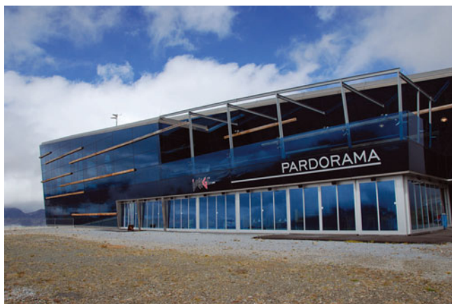
Fig. 11. Mountain restaurant 'Pardorama' in Ischgl, Austrian Alps, located at 2600 m a.s.l. in permafrost terrain. The building weighs 1400 tons. It is underlain by a three-point foundation which can be raised using hydraulic pumps; steel plates can be inserted below to compensate for settlement of the underlying substrate (currently \sim 4 \text{ cm a}^{-1} ). (Photo: M. Phillips 2010.)
