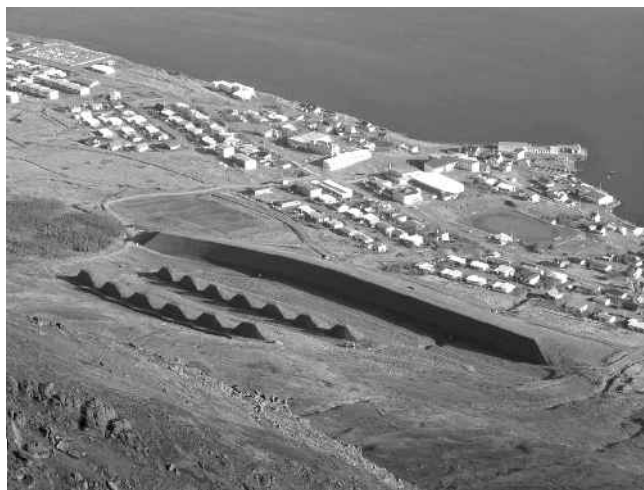
Fig. 1. A photograph of the braking mounds in Neskaupstaður and the catching dam behind them. Each mound is 10 m high, and the catching dam 17 m high.
