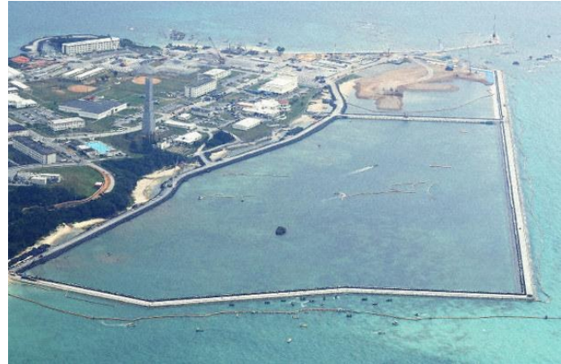
Henoko base construction
