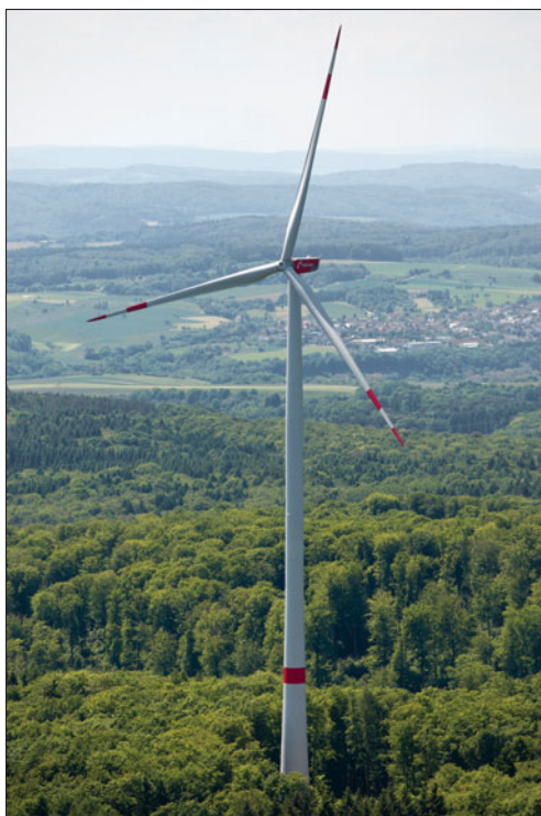
Wind turbine at a wind farm in Hesse, Germany, with a capacity of 2.4 MW (courtesy of Nordex).
