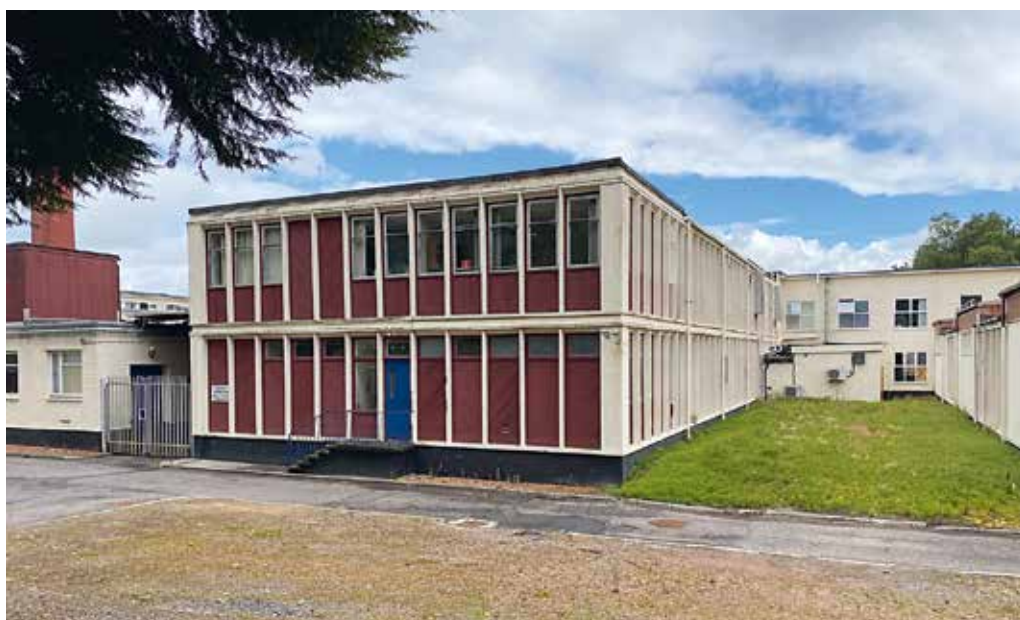
Fig 4. Vale of Leven Hospital, standard unit on west side, formerly laboratories and pharmacy, seen from the west, photograph of 2022 by the author
