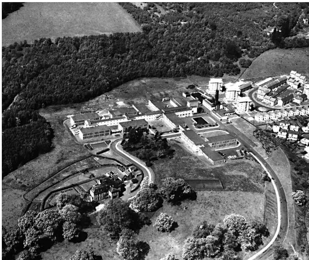
Fig 2. Vale of Leven Hospital, aerial view from the southeast, photograph of 1966 (© courtesy of Historic Environment Scotland, Aerofilms Collection)
