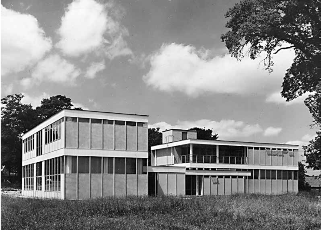
Fig. 12. Clarendon secondary modern school, Oxhey, Hertfordshire, prototype classrooms by Bruce Martin and R. de Yarborough Bateson, 1949–51, photograph of c. 1950 (© Architectural Press Archive / RIBA Collections)
