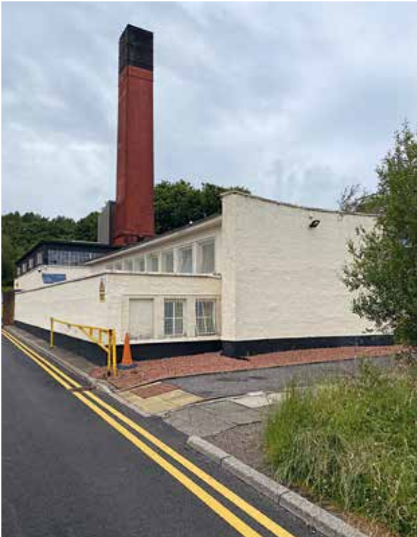
Fig 5. Vale of Leven Hospital, mortuary and boiler house seen from the north, photograph of 2022 by the author
