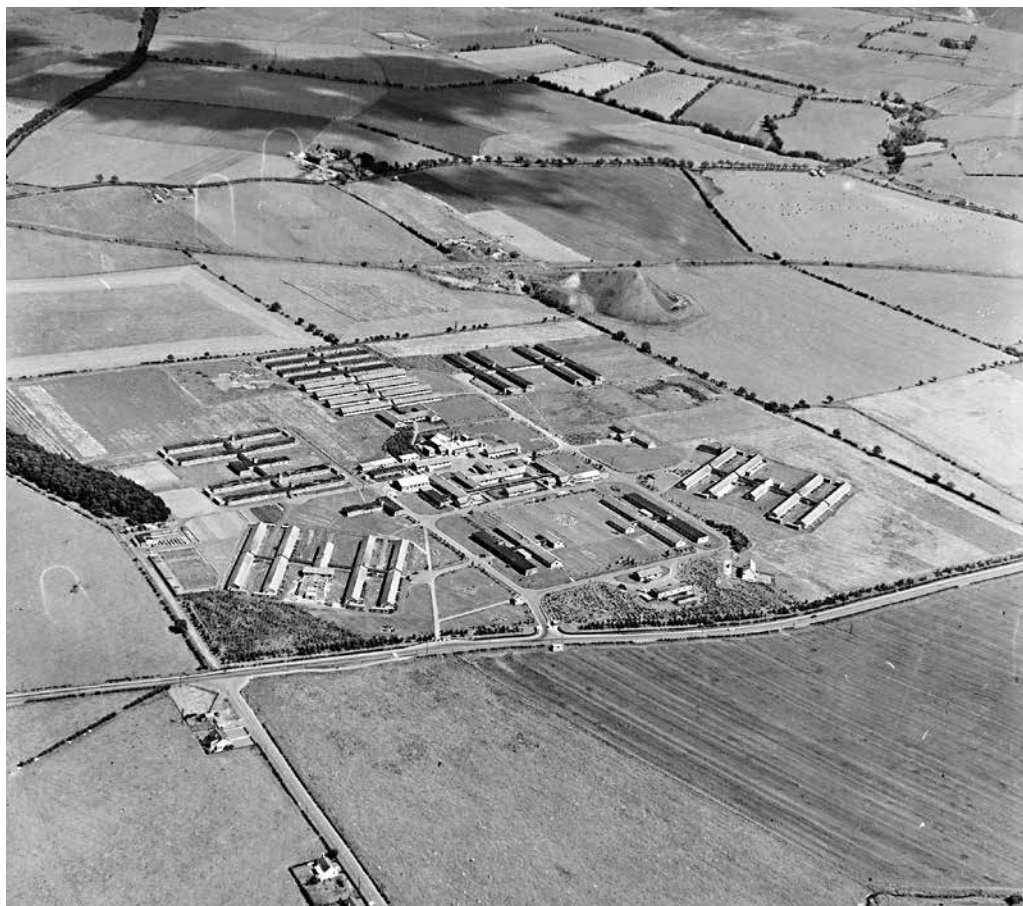
Fig 6. Law Hospital, Carlisle, Lanarkshire, aerial view from the west, photograph of 1953 (© courtesy of Historic Environment Scotland, Aerofilms Collection)
