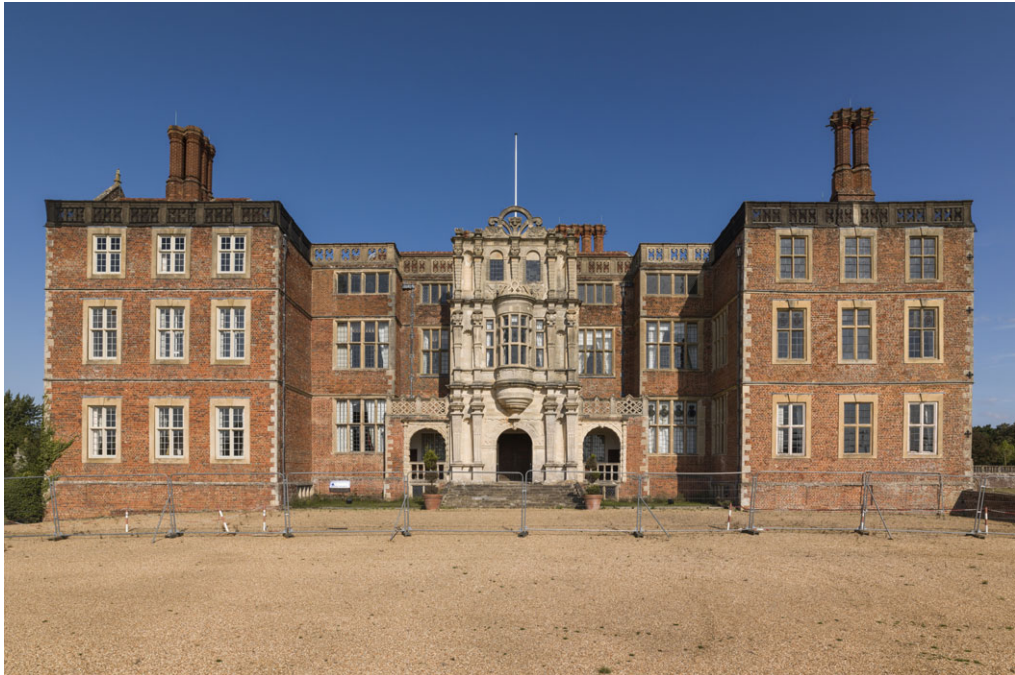
Fig 4. The west elevation of Bramshill in 2016. The stone frontispiece was built in 1612 or shortly afterwards. Wings that originally projected to each side were demolished in about 1703. Photograph: © Historic England Archive, DPI84533, reproduced with permission.
