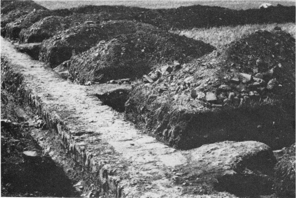
A. Caistor by Norwich: Basilica, west wall of nave looking SW., showing traces of bonding tiles and clunch facing (p. 7).
