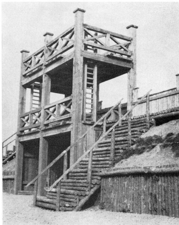
B. The Lunt, Baginton, Warwickshire: experimental reconstruction of east gate of fort on its original site (p. 262).
