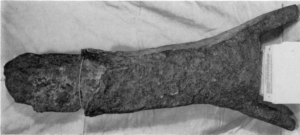
Broken beam from Leicester (3 ft. overall length) showing
