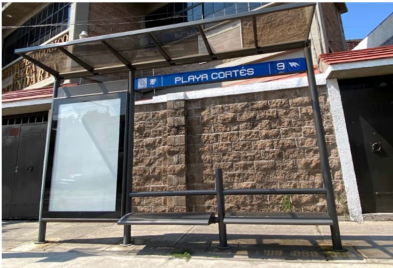
Figure 6. Example of a recently constructed trolley stop. Photo credit: first author, July 2021.
