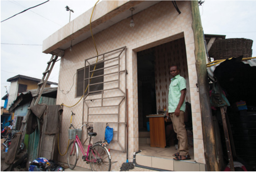
Figure 12 Latrines installed by local sanitation business
