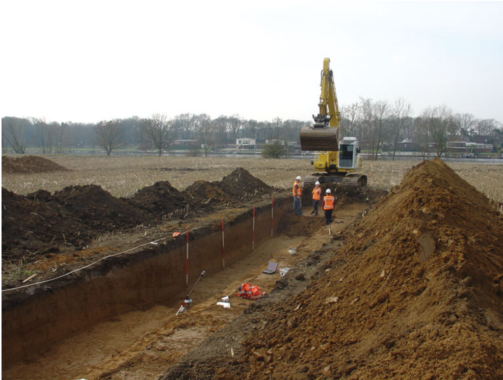
Fig. 1. One of the many trial trenches dug in Well-Aijen, section 2, summer 2011.
