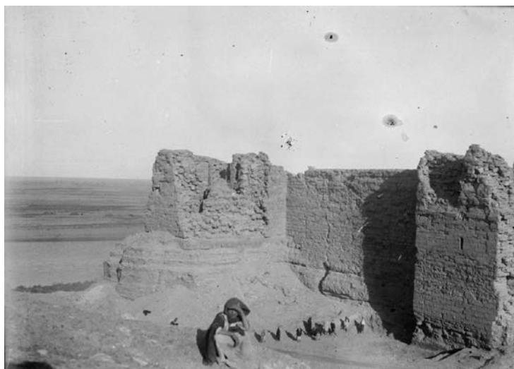
Figure 1.9 Excavations at Dura-Europos: the northern wall of the citadel (1928–9)
