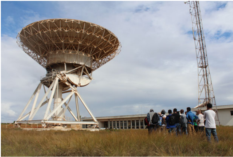
Figure 1. A local Intelsat station to be converted into a radio dish as part of the AVN project.
