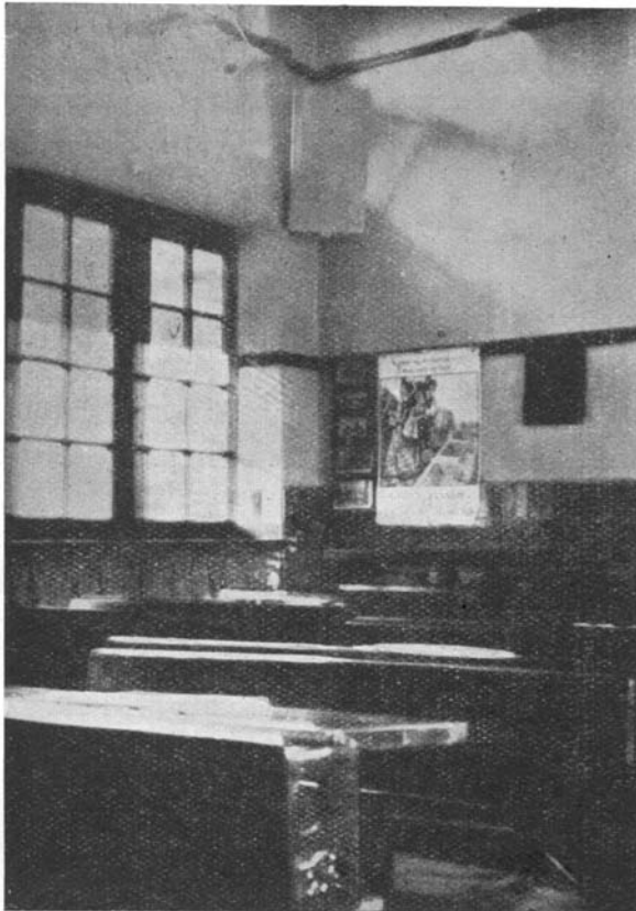
Fig. 1. Photograph of a classroom heated by radiant heat from electric wall panels, one of which is seen in the corner at a height of 7 feet 3 inches above floor level.
