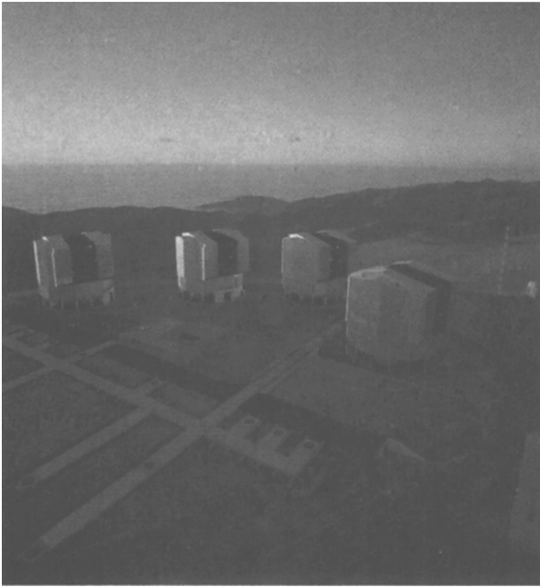
Figure 1. The four 8.2 m telescopes on Paranal, from left to right UT1, UT2, UT3, UT4. Also visible are the stations (holes) where the smaller 1.8 m auxiliary telescopes (ATs) can be positioned. The dark band running left-right shows the position of the underground delay line tunnel. (ESO PR Photo 14a/00)
