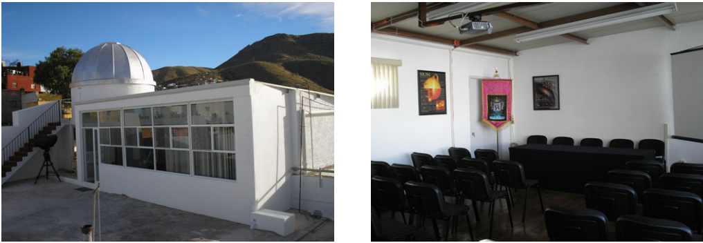
Figure 3. (a) The Observatory after the main reparations were accomplished. (b) View of the room after works and refurbishment.
