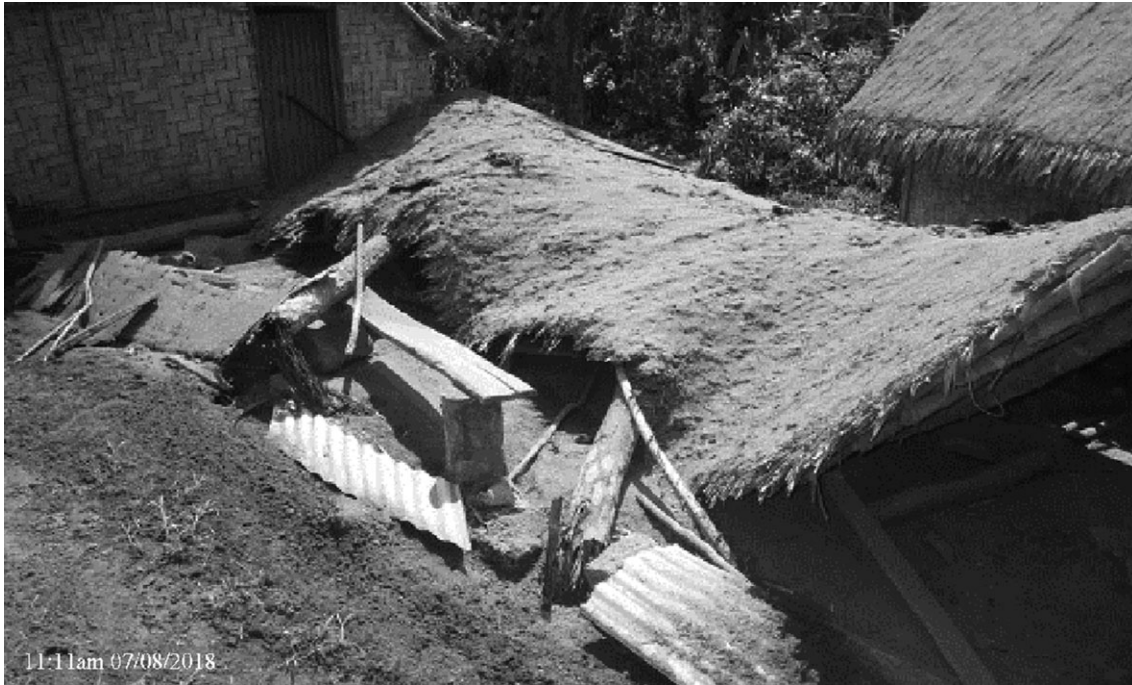
Figure 4. Complete Collapse of an Open-Sided Traditional Building (55mm ashfall depth). Photo Credit: Susannah Jenkins, Earth Observatory of Singapore.
