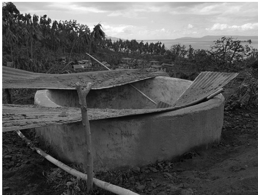
Figure 3. Village Well Contaminated with Ashfall after Protective Metal Sheets Collapsed, South Ambae.
