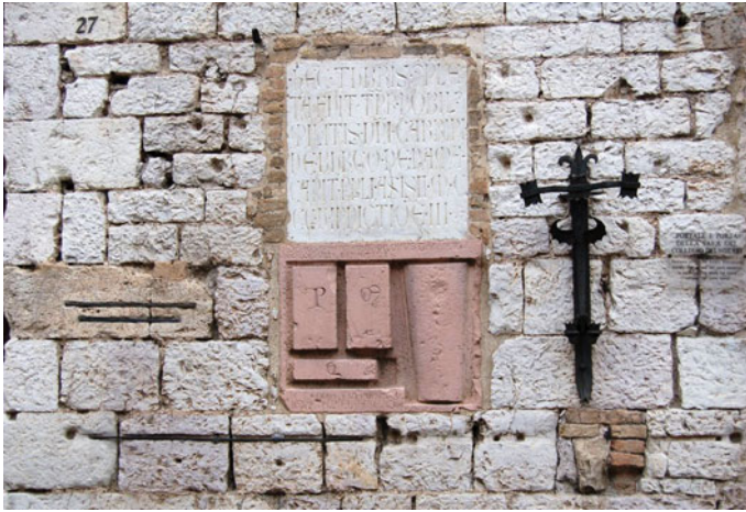
Fig. 5. Assisi, Torre del Popolo, public units of measurement, 1349. Note the three metal rods, at the bottom and left, indicating lengths (canna, passetto, palmo)
