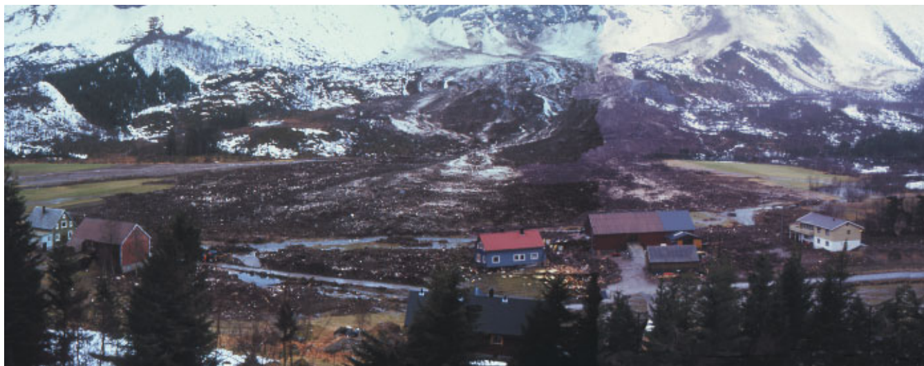
Fig. 1. A huge slushflow released from a low-grade snowfield of high water content on the lower part of the mountain slope has destroyed the farm buildings at Fivelstad, Stranda, West Norway, 5 February 1990. (Photo by K. Kristensen, NGI)
