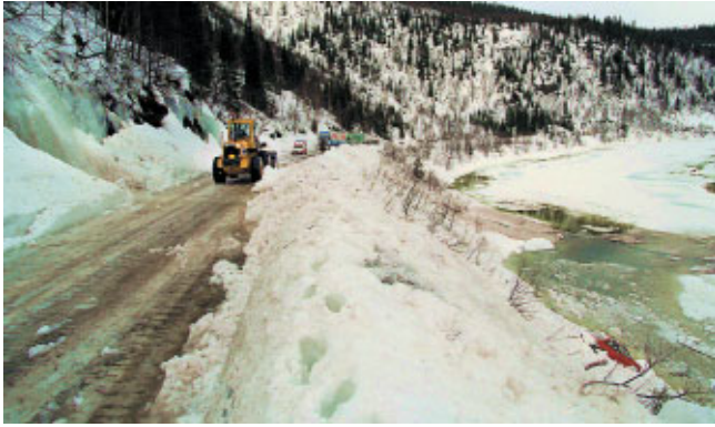
Fig. 4. E6, the main road through North Norway. Six narrow slushflow paths cross the highway within a short distance. Traffic was running freely after the first closure when a flow in the nearest path hit the car, throwing it off the road. Fortunately, the driver escaped unharmed. Illhullia, 26 February 1998. (Photo by Ø. Bratt, Rana Blad.)
