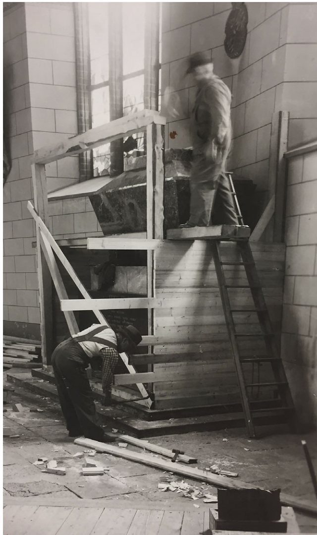
Image 1. A protective structure is being built around the tomb of King Erik XIV in Västerås Cathedral, April 1940. Courtesy of Västmanlands Läns Museum, Vlm-A 658. Photographer unknown.
