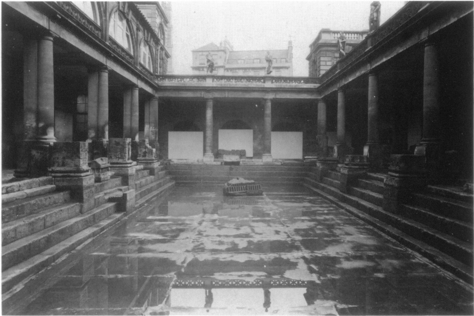
Plate 3. The Great Bath at Bath. In the Roman period the bath was enclosed, and the bases of the piers that supported the massive roof are visible beneath and beside the modern columns. Temporary drainage of the pool reveals its lead-lined floor and stepped seating around the sides. (Photo, Bath Archaeological Trust).
