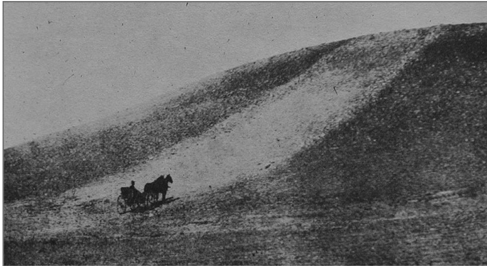
FIGURE 4. The Aztec Airport Mesa Road in 1916. Note the monumental scale and white surface treatment (Wadleigh 1916:52).
