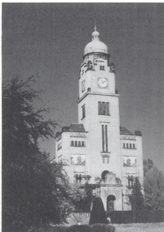
St Venceslas church in the Bohnice hospital: the services restored after more than 40 years of silence
