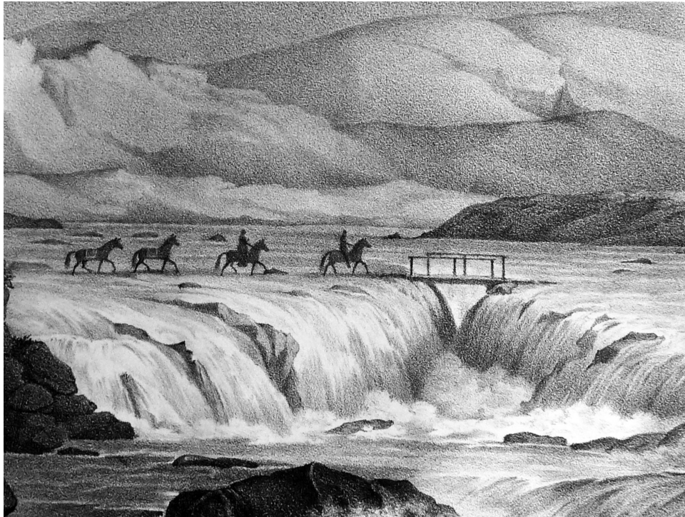
Fig. 3. The bridge over Bruará with the railings that had been added between Irminger's first and second visit. Detail of lithography by Theodor Kloss 1835.
