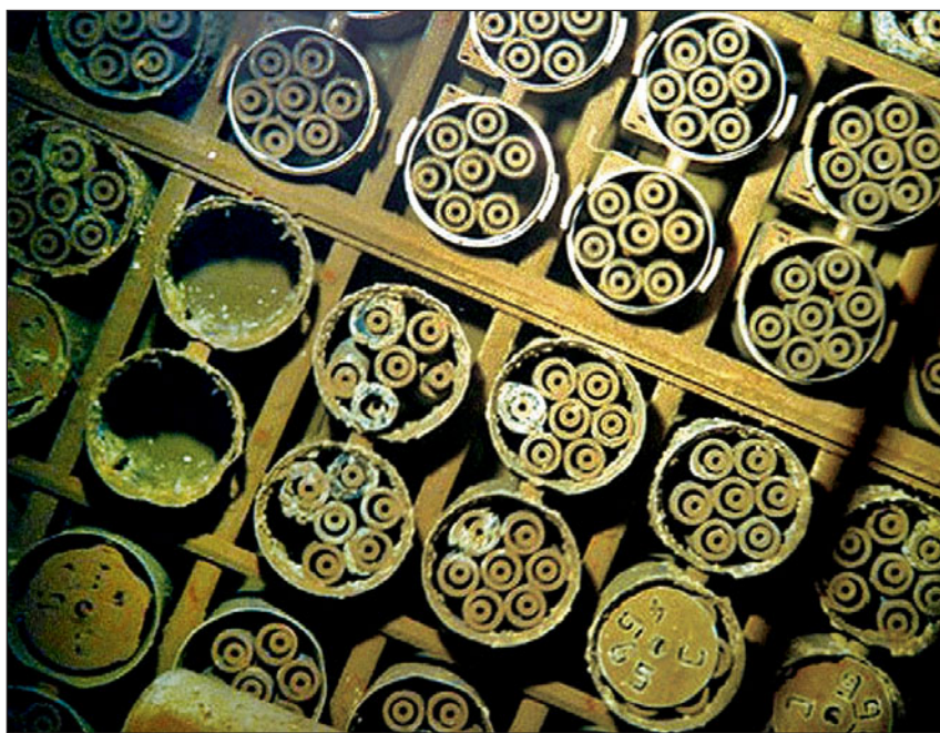
Spent nuclear fuel in uncapped canisters at the US Department of Energy (DOE) Hanford facility in Washington. Credit: DOE.
