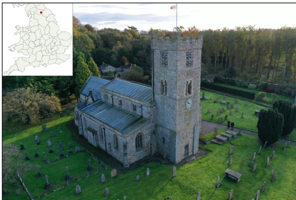
Fig 15. Oblique photograph of St Mary’s Church, Hornby, showing the eleventh-century tower-nave, now integrated as the western tower and (inset) Hornby’s location in central Britain. Image: authors © Crown Copyright and Database Rights. Ordnance Survey (Digimap Licence).
