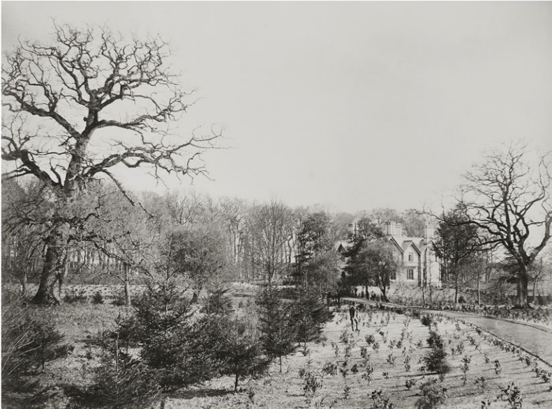
Figure 5. 1865 photograph showing Bachelors' cottage. In twenty years' time, the trees would become thick with conifers, which provided a screening effect, shielding the estate from nearby roads. Source: Royal Collection Trust.
