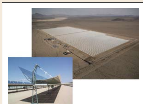
Figure 1. Aerial photograph of Acciona's Nevada Solar One, a 64 MW parabolic trough power plant near Las Vegas, Nevada, that covers 280 acres (Credit: Acciona Solar Power). Inset: Closeup of an individual parabolic trough unit at Kramer Junction, California, showing the curved mirror and the receiver (Credit: Henry Price).
