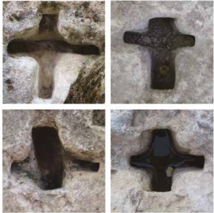
Fig. 15. Ancient blocks with superimposed lewis cuttings from different phases of construction, photographs by Philip Stinson (courtesy of the New York University Aphrodisias Excavations)
