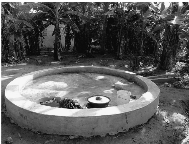
Fig. 4. Newly installed washing platform.
