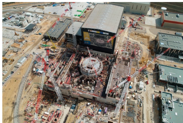
Figure 9. Bird's eye view of the ITER site in Cadarache with the growing torus hall in the middle; status: March 2018 (courtesy: ITER Organization/EJF Riche; more photos available under: https://www.iter.org/album/Media/4%20-%20Aerial ).
