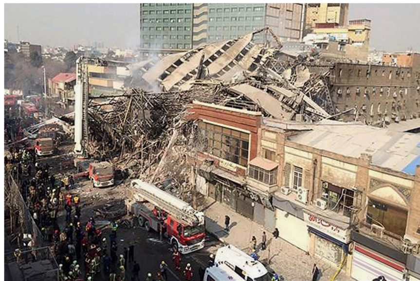
View of Plasco Building Collapse Scene.
