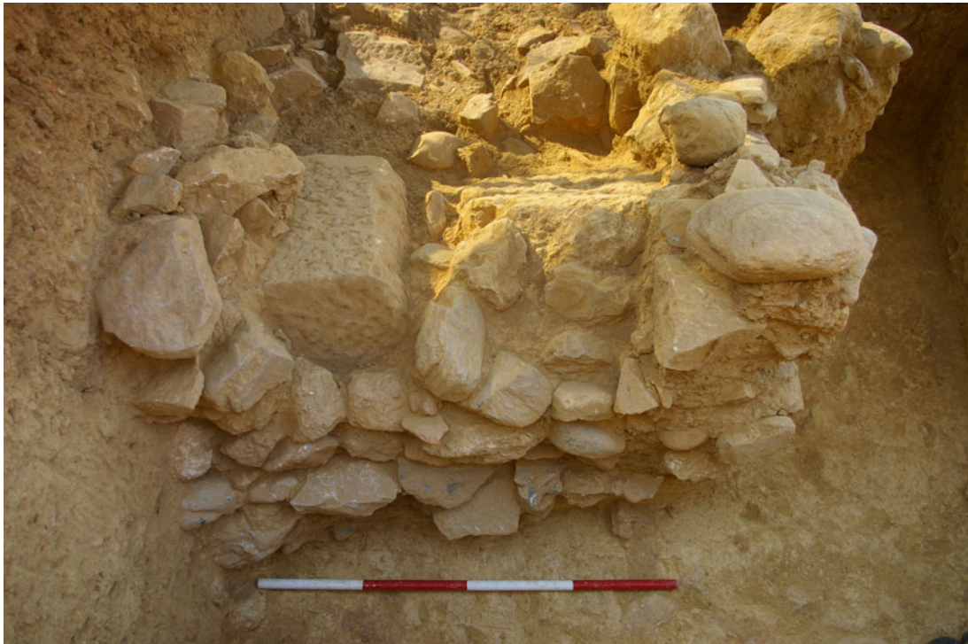
Fig. 2.13. Northern elevation of terrace wall in C513 in Trench 2. Note the large block of worked stone in the centre left of the image.
