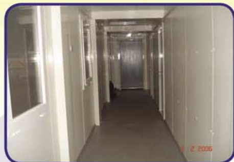
Inside MSF Hospital in Hattian Bala
