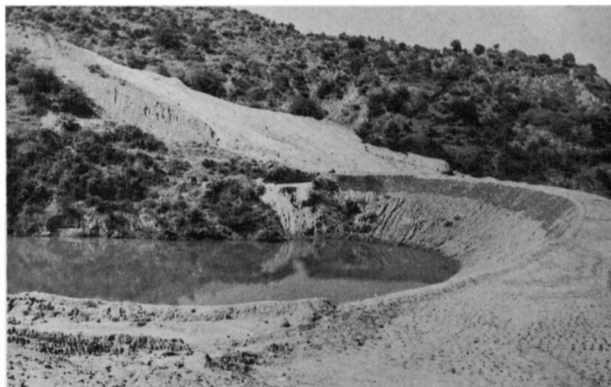
FIG. 3. Another Sukhomajri check-dam reservoir with, behind, a revegetated hill that at one time was practically barren.
