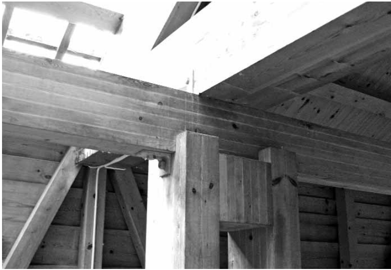
The structure brought to the light, Hedmark Cathedral Museum, Hamar (1979) 2
