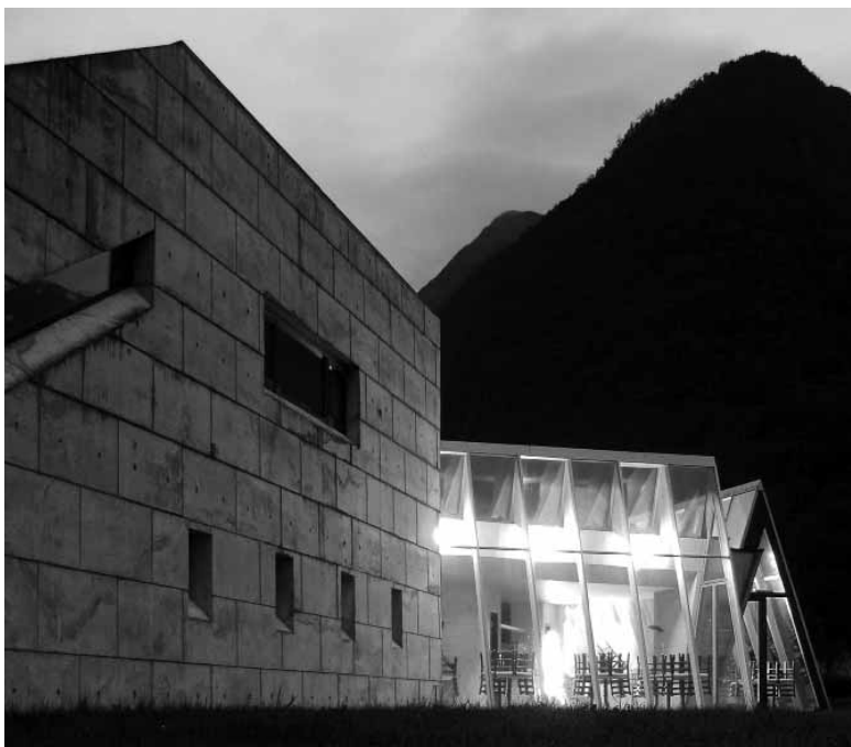
The construction as a microcosm of the site: the Glacier Museum, Fjærland (1991) 4
