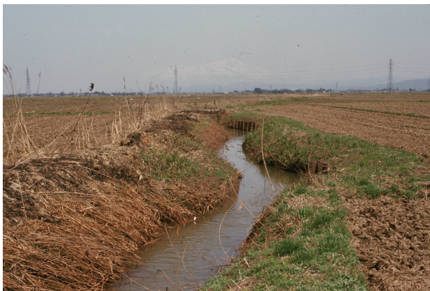
An old unlined branch canal
