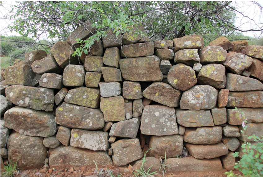
Figure 3. Remains of drystone walling at Marothodi: a) Collapsed walls surrounding a central cattle enclosure; and b) detail showing the construction of drystone walling (photographs by P.D. Fredriksen).
