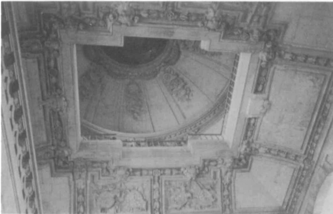
Fig. 14. François Mansart. Blois, Orléans wing. Staircase roof
