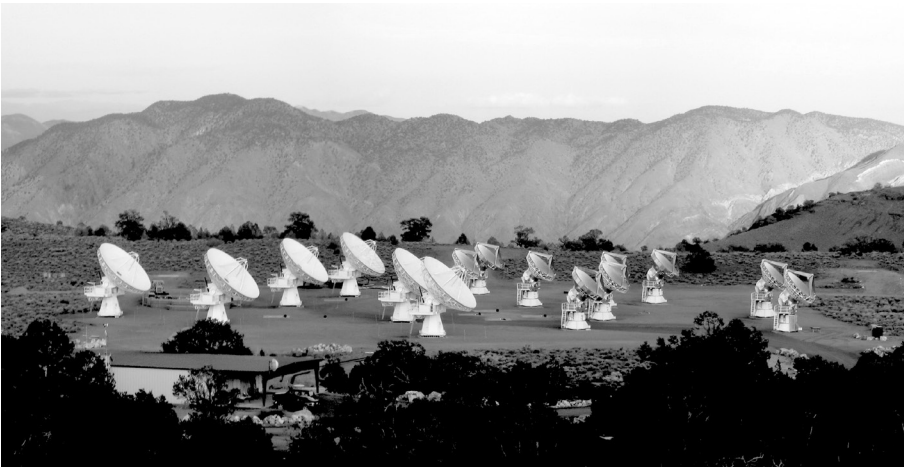
Figure 2.4 CARMA: six OVRO 10.4 m antennas on the left and nine BIMA 10 m antennas to the right. Courtesy of Anneila Sargent, reproduced by permission.
