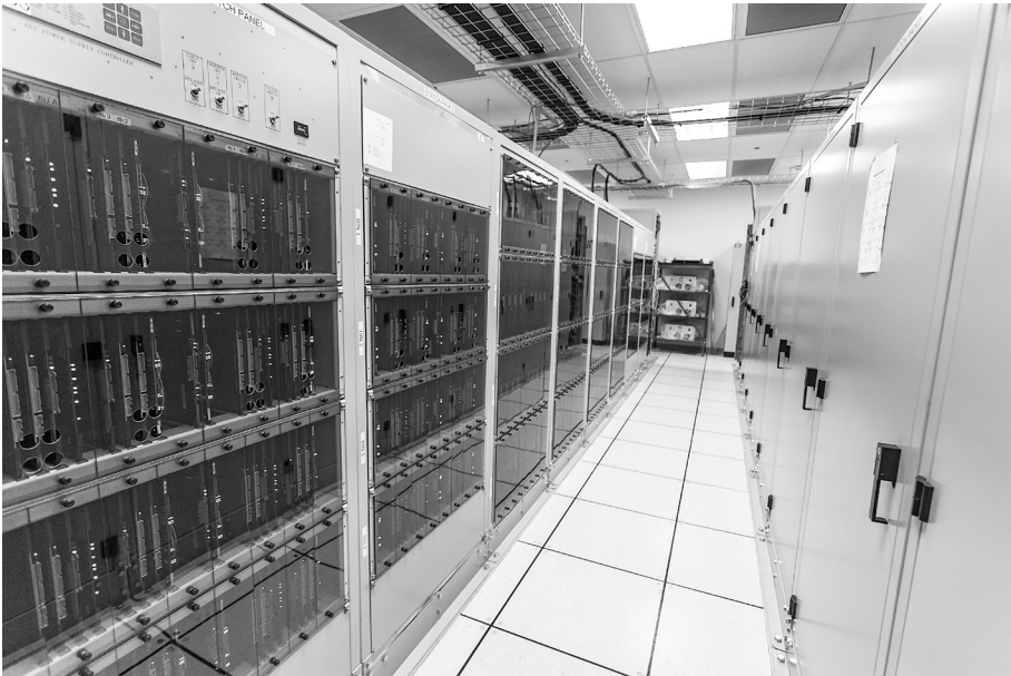
Figure 9.11 View along the rack fronts of one quadrant of the correlator for the 12 m antenna array, located in the ALMA Technical Building at 5,000 m above sea level. Credit: ALMA/ESO/AUI/NINS, CC BY 4.0.
