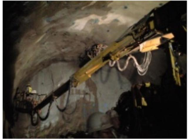
**Fig. B1.** The drilling machine in use at a tunnel construction site.
