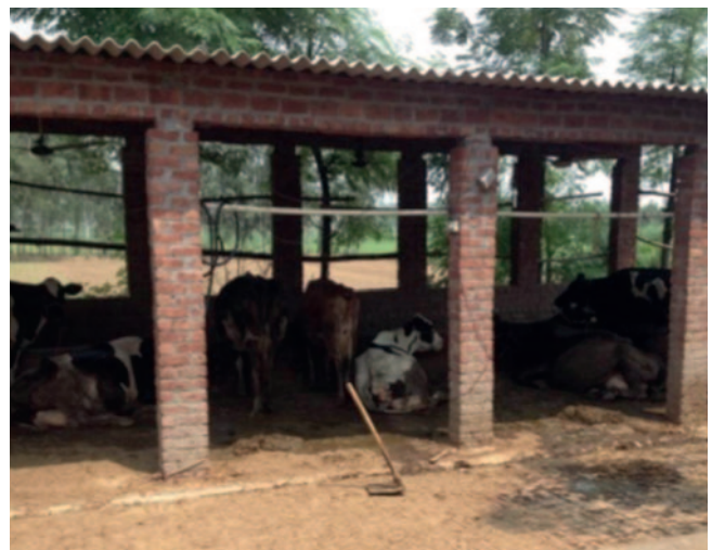
Loose-housing system with brick-on-edge flooring and use of ceiling fans for protection against heat stress at a medium farm.
