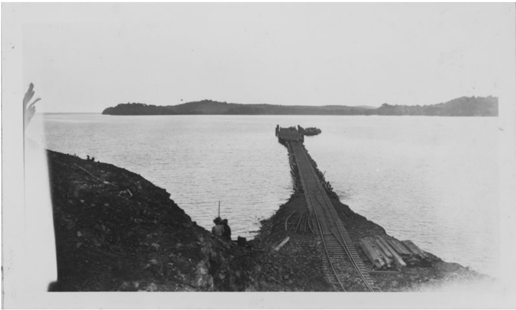
Figure 5. The rail platform pier allowed products to be loaded onto large cargo ships. The pier is still in use but is now paved over.
