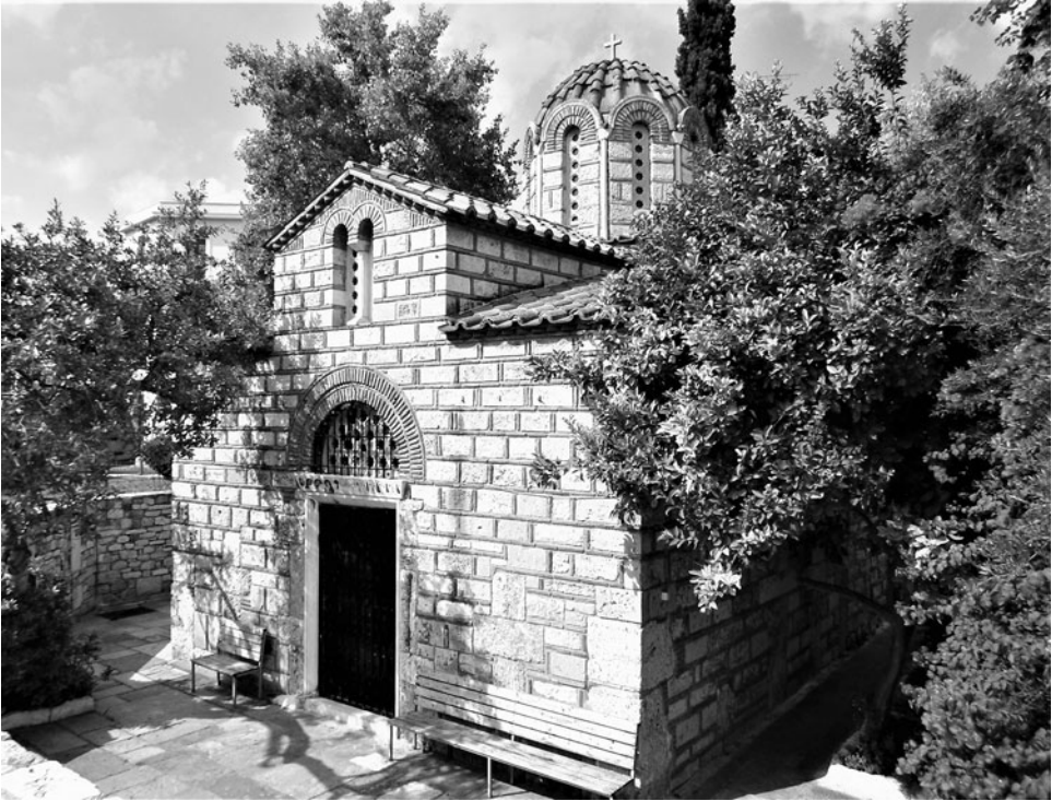
Fig. 3. The eleventh century Agioi Asomatoi at Thiseio as seen today. In the late nineteenth century it was greatly enlarged and an elaborate bell tower was added at its west side. Between 1959 and 1960, restoration projects by the Directorate of Restoration reinstated the monument to its original Byzantine size and form. Photograph by the author.
