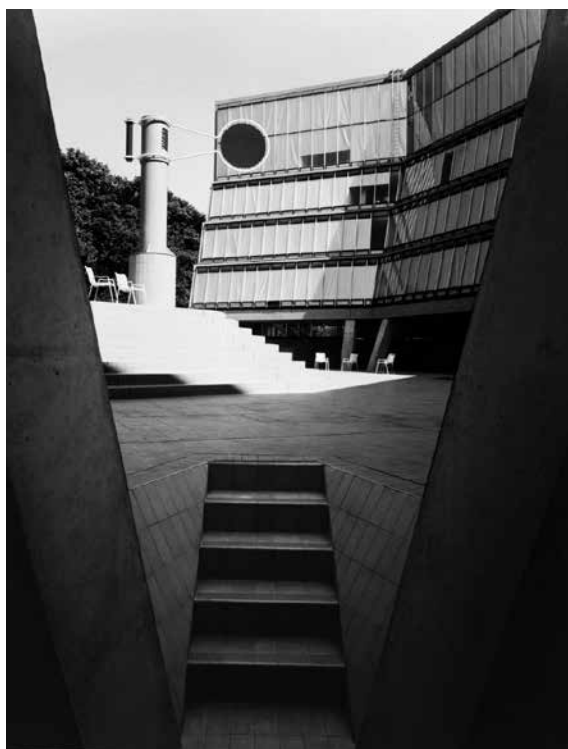
3 Exterior view of James Stirling's Florey Building, Queen's College, University of Oxford (Oxford) between 1966 and 1971, gelatin silver print, 25.4 x 20.3 cm. Ironically placed on a functional 'pedestal', the kitchen fan alludes to the founder's bust
