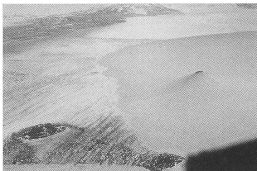
Fig. 8. Aerial photograph taken in November 1980 showing the ice edge looking south and to the rear of the easternmost Dailey Islands. Brown Peninsula is at the top left of the photograph. Koettlitz Glacier is located at the top right.
