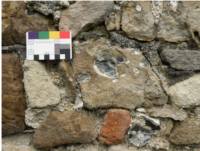
Fig 2. Sarsen in the walls of St Peter's church, Broad Hinton (Wiltshire), demonstrates the variability both of its use – here as rubble walling rather than cut blocks – and its lithology, with flint pebble clasts amongst the cemented sand in some pieces. Photograph: the author.
